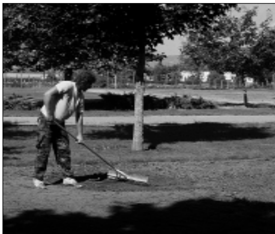
Figures 2 and 3.—After tilling, use a water-filled roller and grading rakes to level and firm the area. Be prepared to go over the area repeatedly to achieve uniform compaction. Grade edges level with concrete surfaces.
