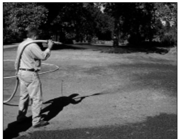
Figure 8.—Hydroseeding applies seed, fertilizer, and mulch all in one operation.
