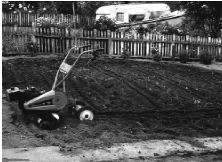
Figure 1.—Rototilling loosens and mixes soil so it can be graded smooth. Avoid overtilling, which can destroy soil structure and cause rapid, excess compaction.
