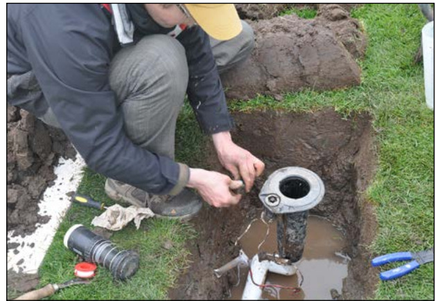
Figure 7. Automatic control irrigation systems typically will have wiring to each irrigation head, or a block of irrigation heads, to provide more precise irrigation.
