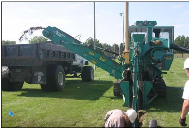
Figure 3: Drainage trenches (6 to 8 inches wide) being cut using a laser-controlled machine.
