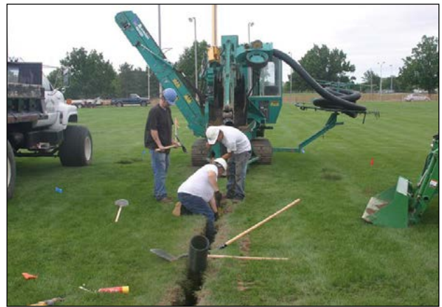
Figure 3: Drainage trenches (6 to 8 inches wide) being cut using a laser-controlled machine.
